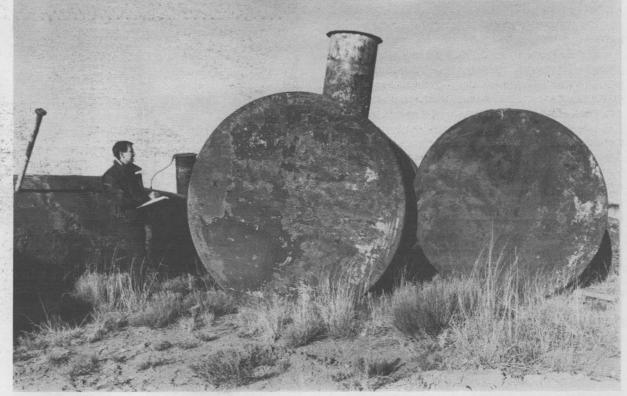
TRACKING TANKS — In this 1989 photo, Sandian Dave Dionne checks the condition of underground storage tanks removed in late 1988. Acccording to state and federal requirements, all USTs must be accounted for, brought into compliance with new regulations, closed in place, or removed by December 1998. (Photo by Randy Montoya)
